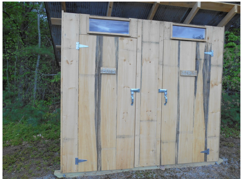
New composting outhouse at the Historical Society School House
